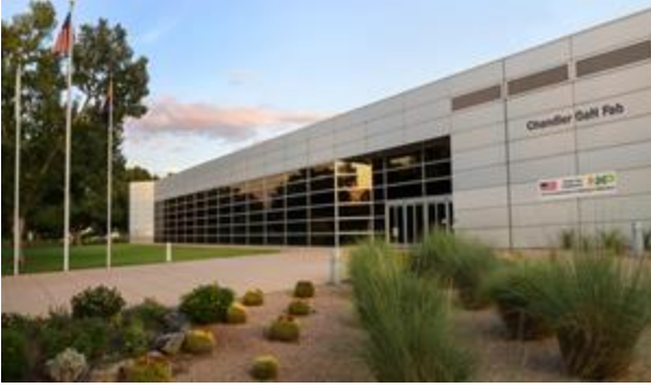
High-volume manufacturing facility is the most advanced GaN fab for RF in the United States
